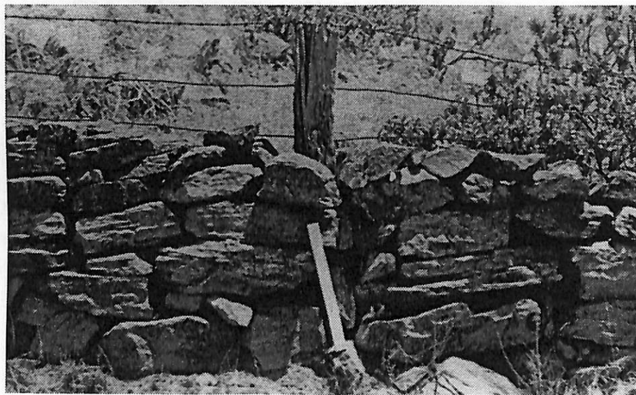
Dry stone wall, Barossa Valley South Australia. 50 cm measure in centre.
