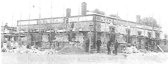
The Blyth Hotel refurbishment under way in 1911.
