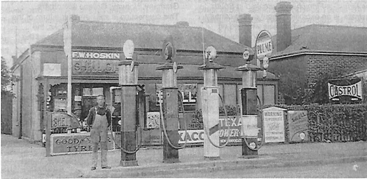
Above: Frank Hoskin's petrol station, South Road. circa WW2.
