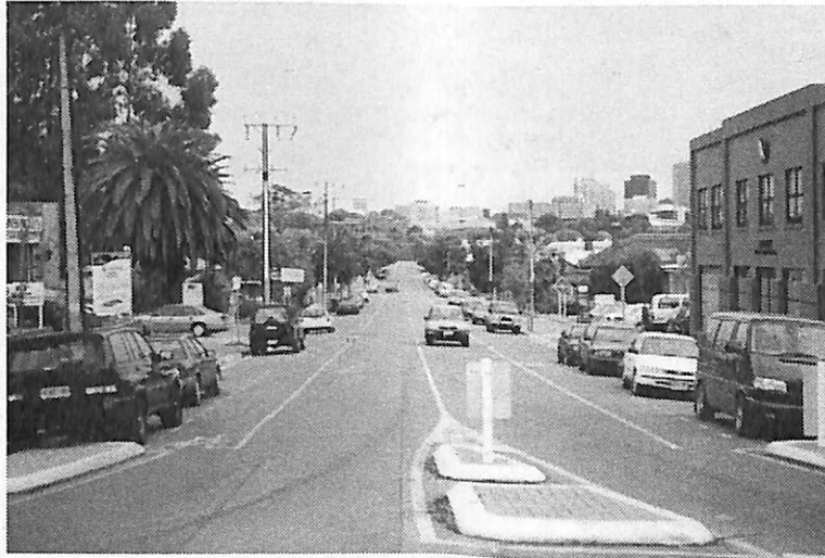
The extensive dip in King William Street, Kent Town, revealing the former path of First Creek.
