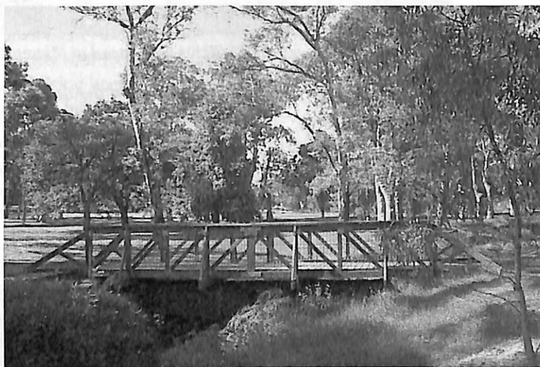
A present-day bridge "in the American fashion" in the east parklands.
