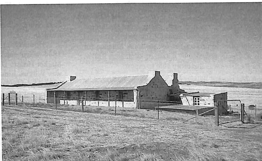
The restored Wilkins homestead at Mount Bryan East.
