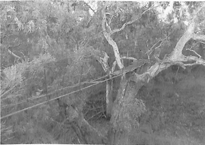
Swing bridge at Lower Light.
