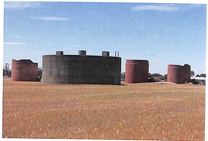
Aviation fuel tanks at Wolseley.
