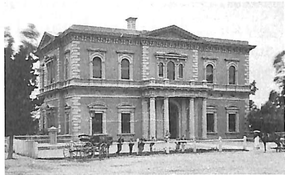
The original 1860 SA Institute Building in 1875. It comprises the southern half of the present building. Image courtesy of SLSA: B10391
