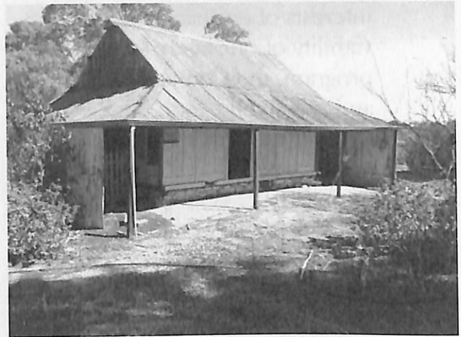
A Manning cottage at Seppeltsfield
