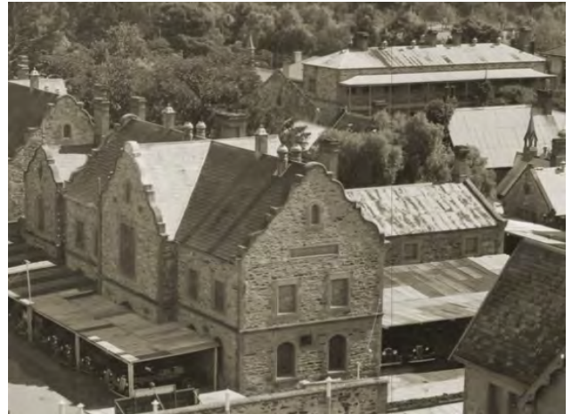
The northern part of the former Destitute Asylum. The vehicles garaged around the men’s infirmary (formerly the Colonial Store) show the small scale of the two-storey building. The lying-in home, now housing the Migration Museum, is top right. By Henry Krischock, 1936 SLSA, B 9360 (cropped)
